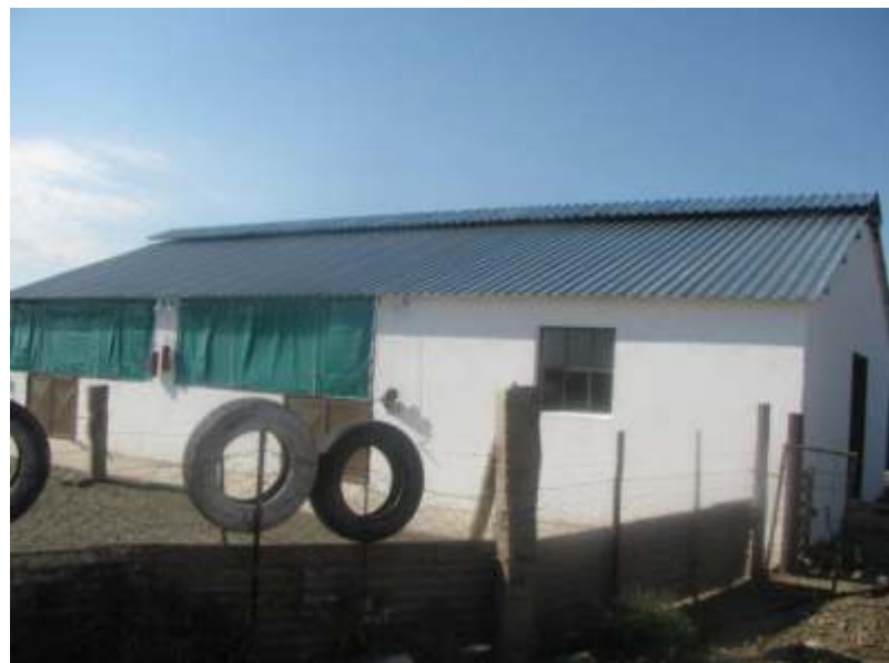
Proper housing structure for raising day old ostrich chicks constructed by the department
