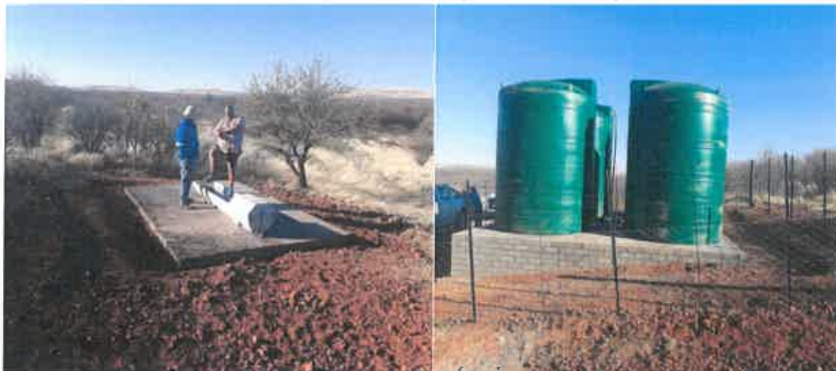
Installation of stock water system at Koopman Farm In Pixley Ka Seme
