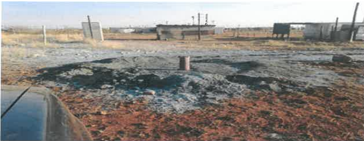
Pictures of the drilling of the boreholes
