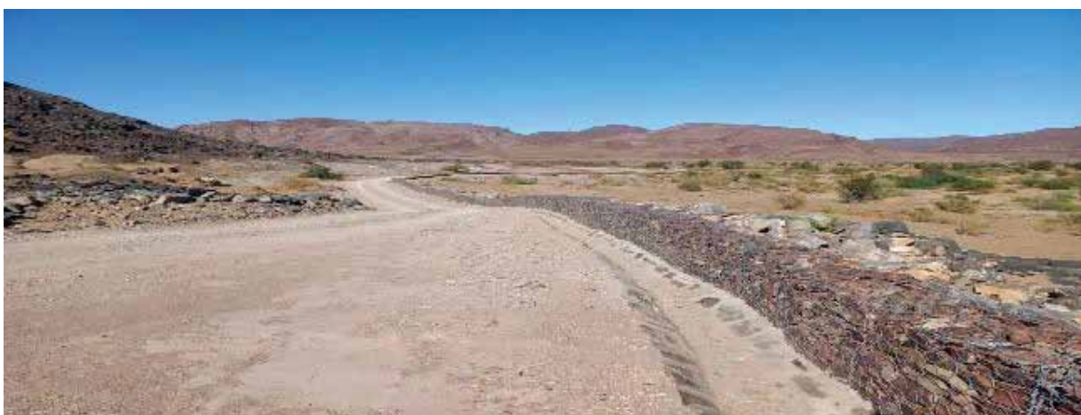
Road had been sloped with stormwater channel with gabion barriers that were constructed at Nababiep Project.
