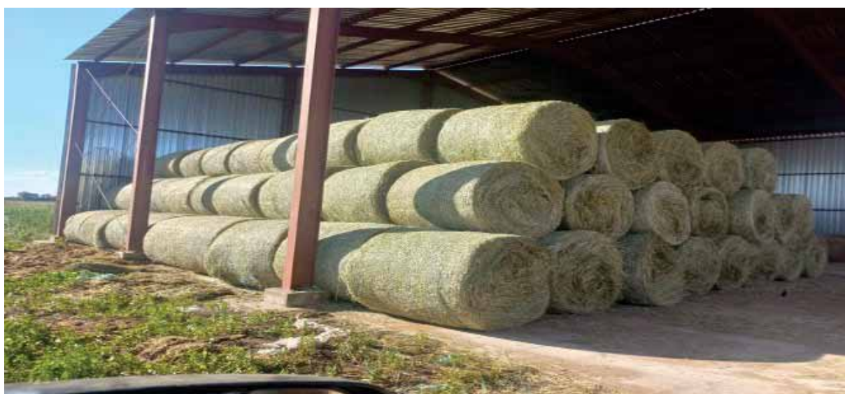
Fodder storage facility showing the open sides exposing it to rain
